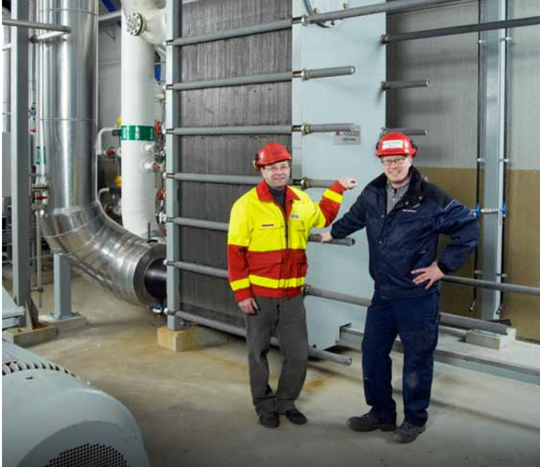
Juhani Sirviö of SYSAV (left) with Sven Brantebäck of Götaverken Miljö AB and the Tranter PHE Model GXD-205 that transfers heat energy from top stage scrubber condensate to district heating water.
