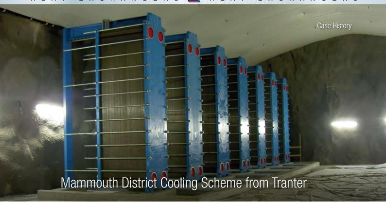
Tranter International AB has demonstrated its experience in the field of district cooling projects with the design and delivery of seven impressively large plate heat exchangers (PHE) with a physical height of around 5 meters each, and total cooling effect of 84 MW. The units are currently being delivered to a project Fortum is carrying
