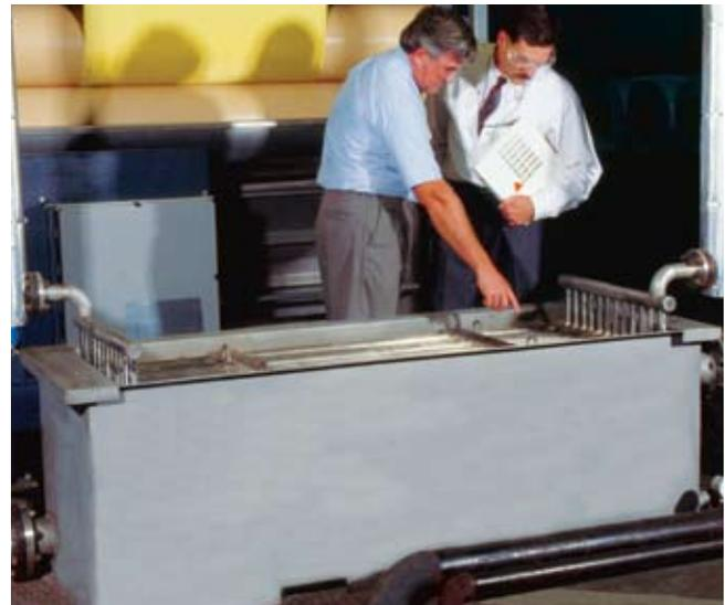
Overflow hot water from three washers (in background) enters the PLATECOIL bank at lower left at 90°C (195°F), then transfers heat to fresh water before exiting to an outside drain (bottom right) at 57°C (135°F).
