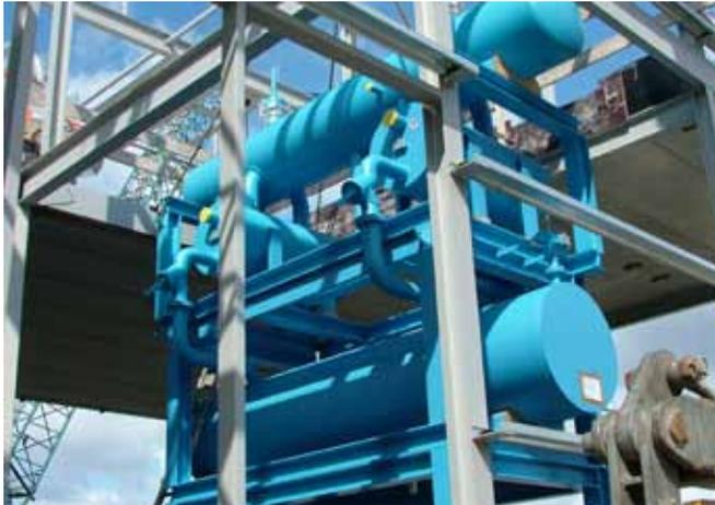
From top: NH<sub>3</sub> separator, two SUPERMAX NH<sub>3</sub>-CO<sub>2</sub> cascade HEs and CO<sub>2</sub> vessel with SUPERMAX cooler.
